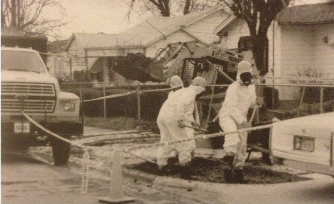
FIGURE 10: Crew cleans up lead-tainted soil in West Dallas, Texas
