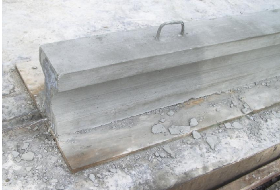
Figure 39. End of prestressed beam before steel strands were torch cut
