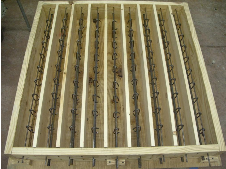
Figure 22. Forms for remaining flexural beams
