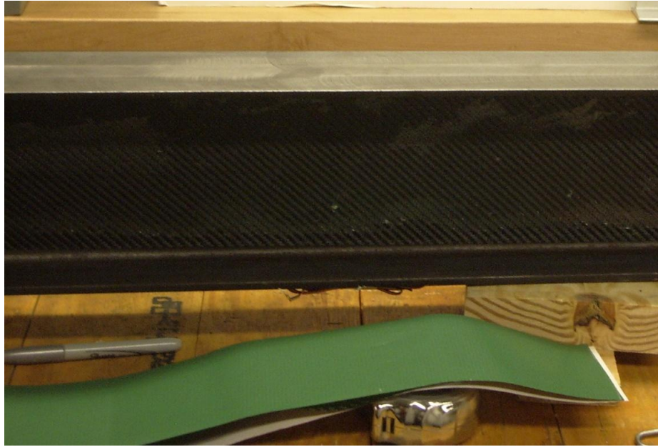
Figure 85. Completed steel web application of LTC 4300
