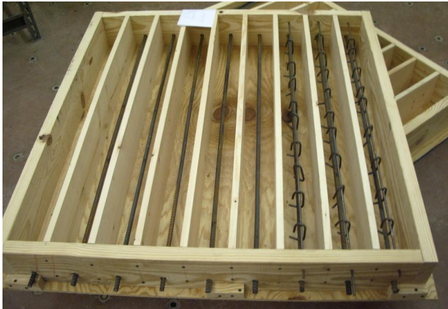
Figure 21. Forms for 6 shear beams and 3 flexural beams
