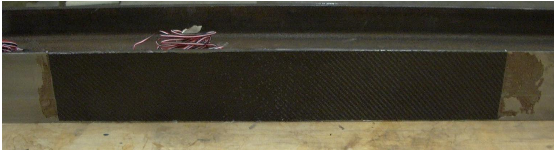
Figure 84. Completed LTC 4300 application to bottom flange
