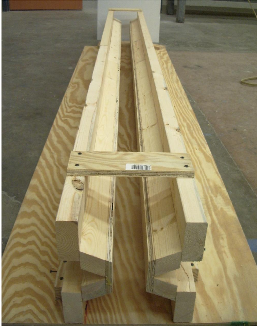
Figure 38. Formwork for prestressed concrete beams
