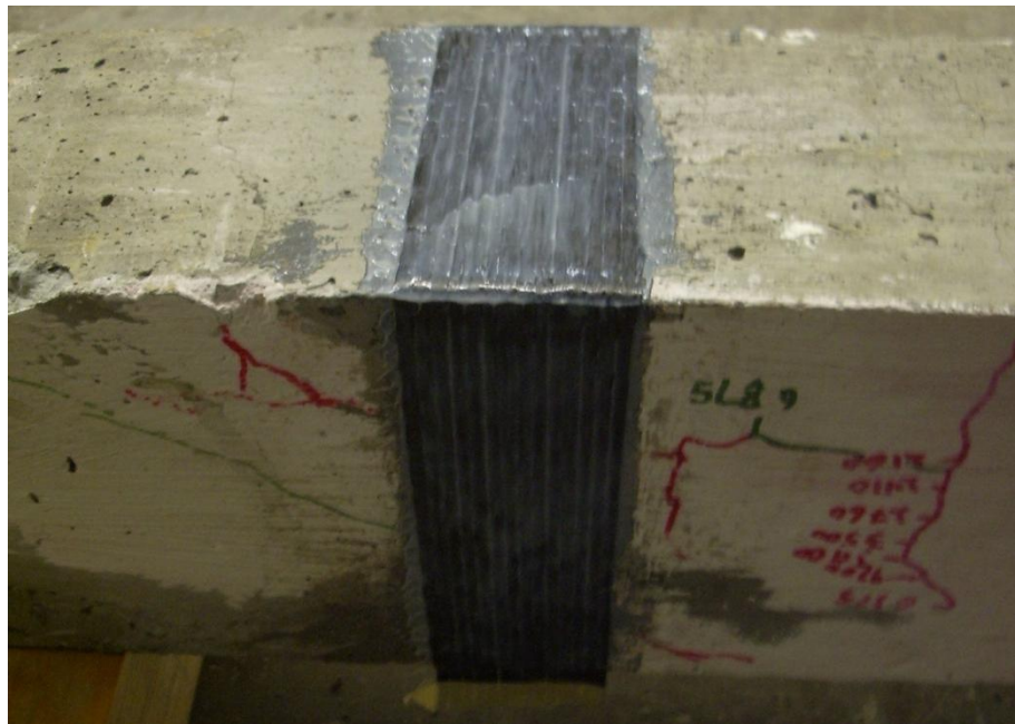
Figure 71. Close up view of Sikawrap reinforcement crossing shear cracks
