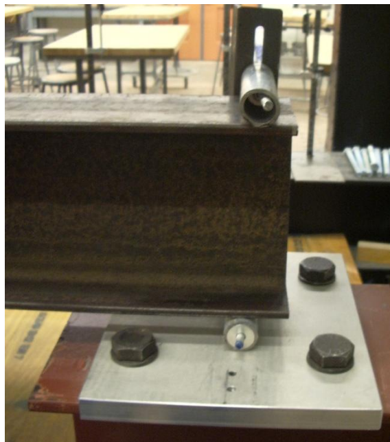
Figure 93. Exposed bearing pins with one lateral brace removed
