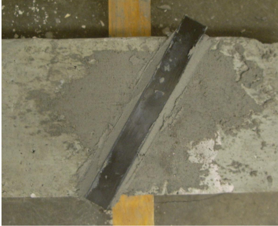
Figure 74. Completed Carbodur shear reinforcement
