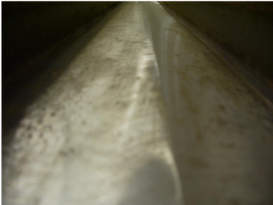
Figure 33. Close up view of milled web of beam SBII, side 2
