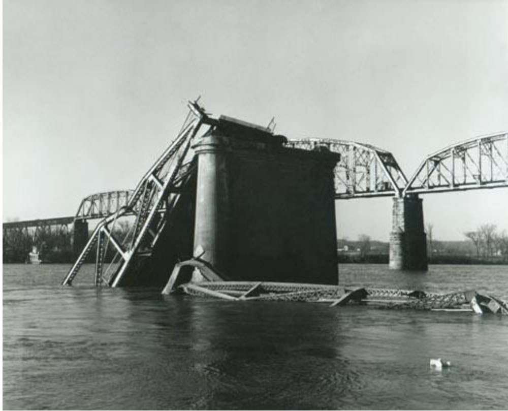
Figure 3. Collapse of Silver Bridge in 1967, caused by fatigue failure of eye bar pin
