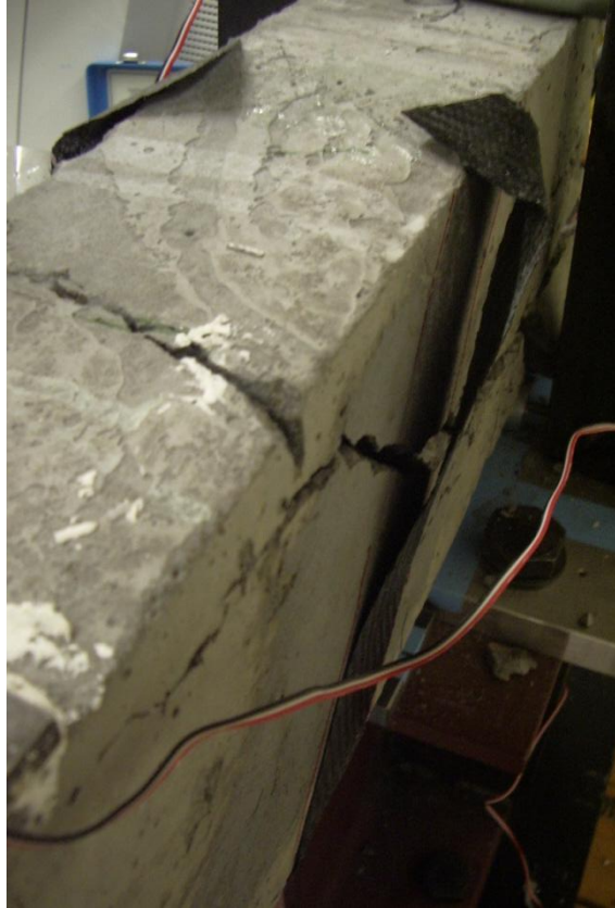
Figure 162. Close up of LTC 4300 debonding
