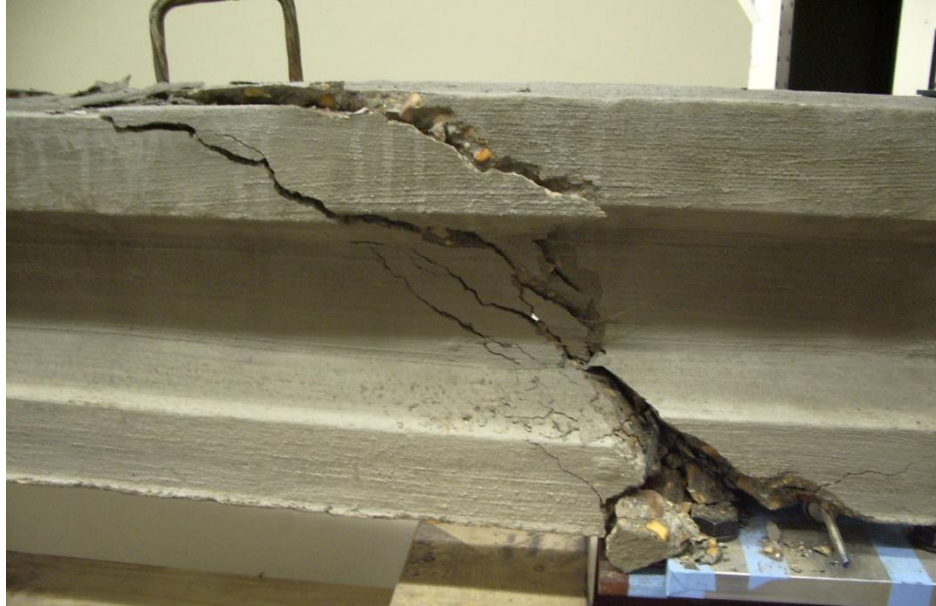
Figure 132. Ultimate shear failure of PSCB2
