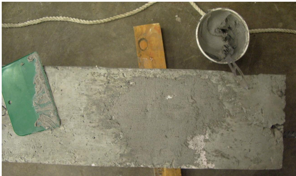
Figure 64. Identical surface repaired with epoxy grout
