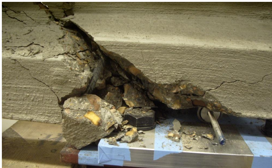
Figure 133. Close up of shear failure of PSCB2, note rebar stirrup
