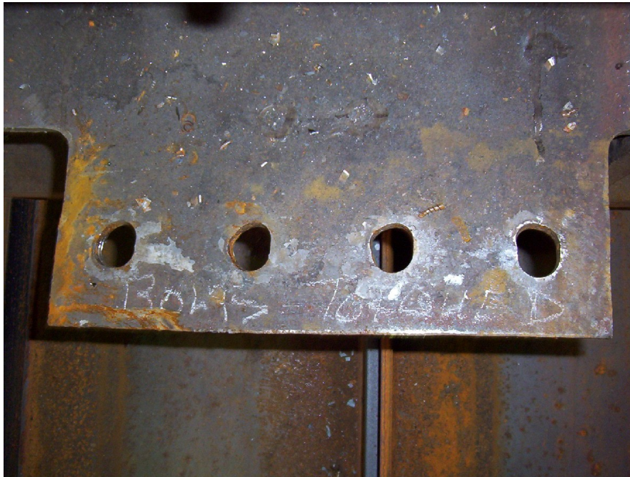
Figure 23: The shear tab holes of test 1-1 after testing
