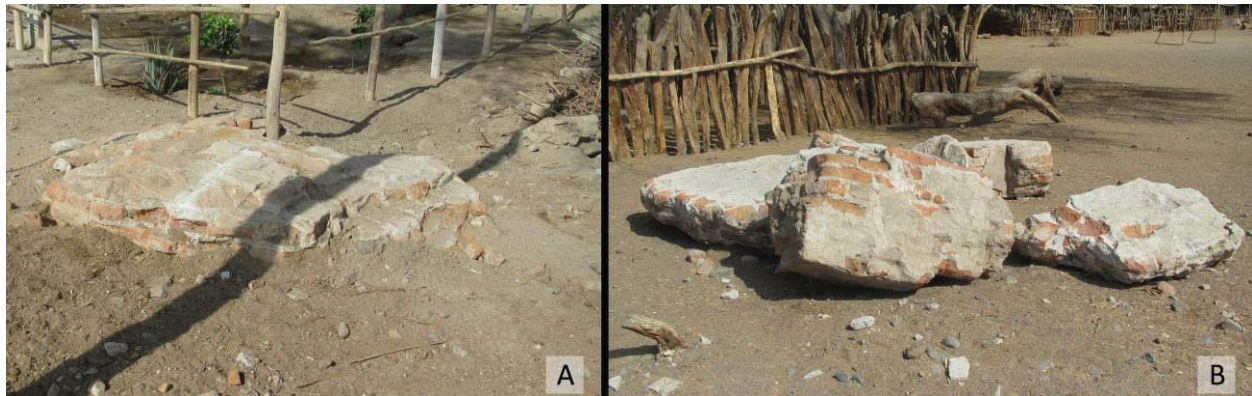
Figure 6.8. Northern hacienda wall at San Xavier. A: extant corner of brick and lime wall. B: portions of the northern hacienda wall that have been hauled to the area south of the community soccer field.
