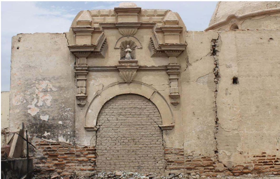
Figure 6.11. Western face of the Jesuit West Gate at San Xavier.
