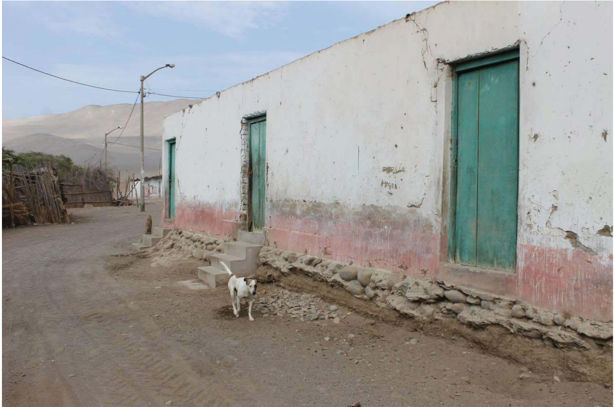
Figure 7.35. One of the few modern residential structures at Coyungo with historical (possibly colonial) foundations.
