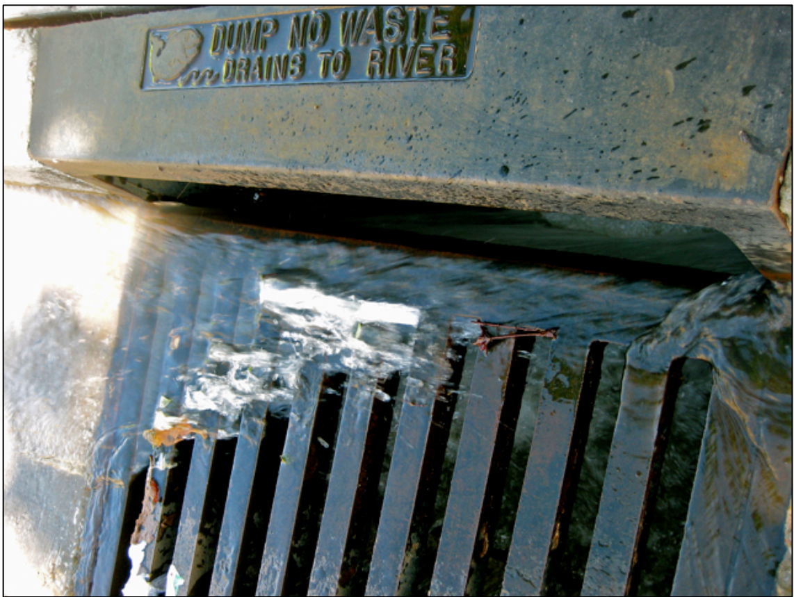
Figure 32. Water rushing into a stormdrain in downtown Nashville. (photo by Jennifer Mokos)
