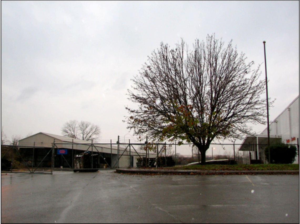
Figure 33. Industrial development hides much of the east bank of the Cumberland River from view. ( photo by Jennifer Mokos )
