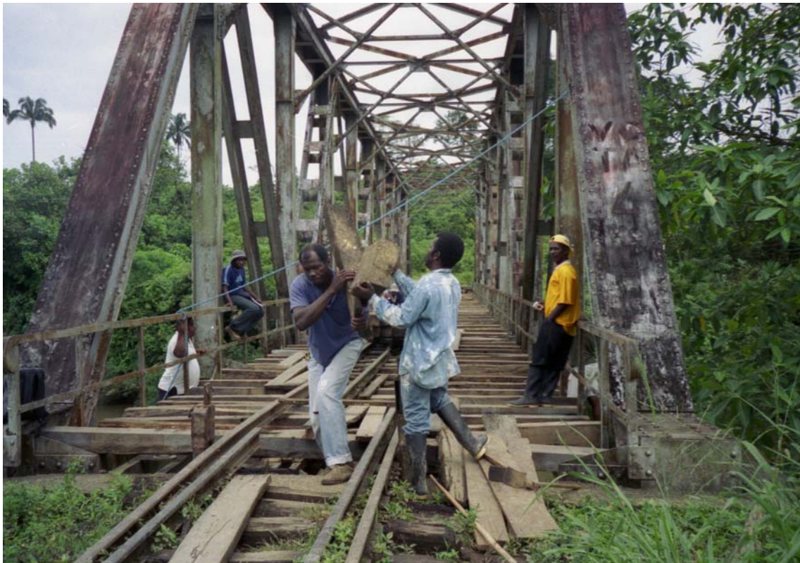
Figure 14. Local employees of a palm plantation turn an unused rail bridge into a bridge that will carry the heavy trucks that transport palm oil fruit to the local refinery. July 2007.
