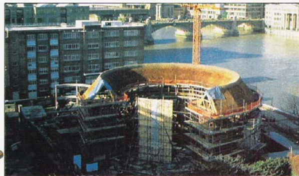
The new Globe Theatre under construction in London.
