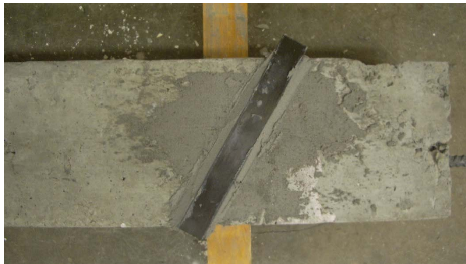
Figure G.2. Shear reinforced concrete beam repaired with FRP composite reinforcement.
