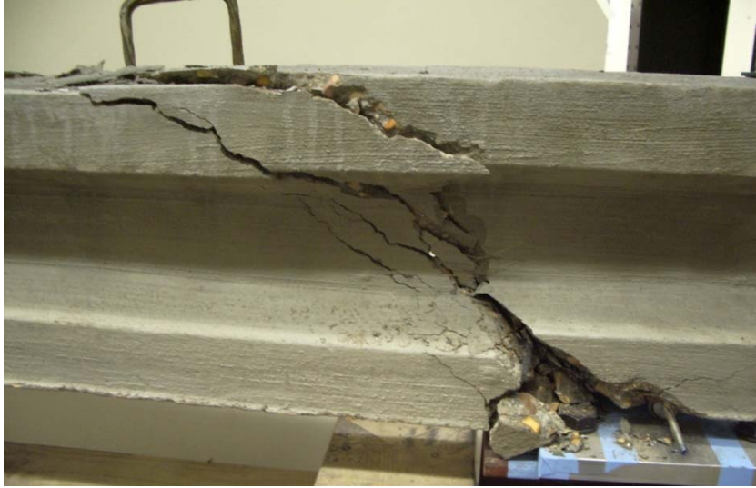
Figure 3.4.23. Ultimate shear failure of the beam PSCB2 [65].
