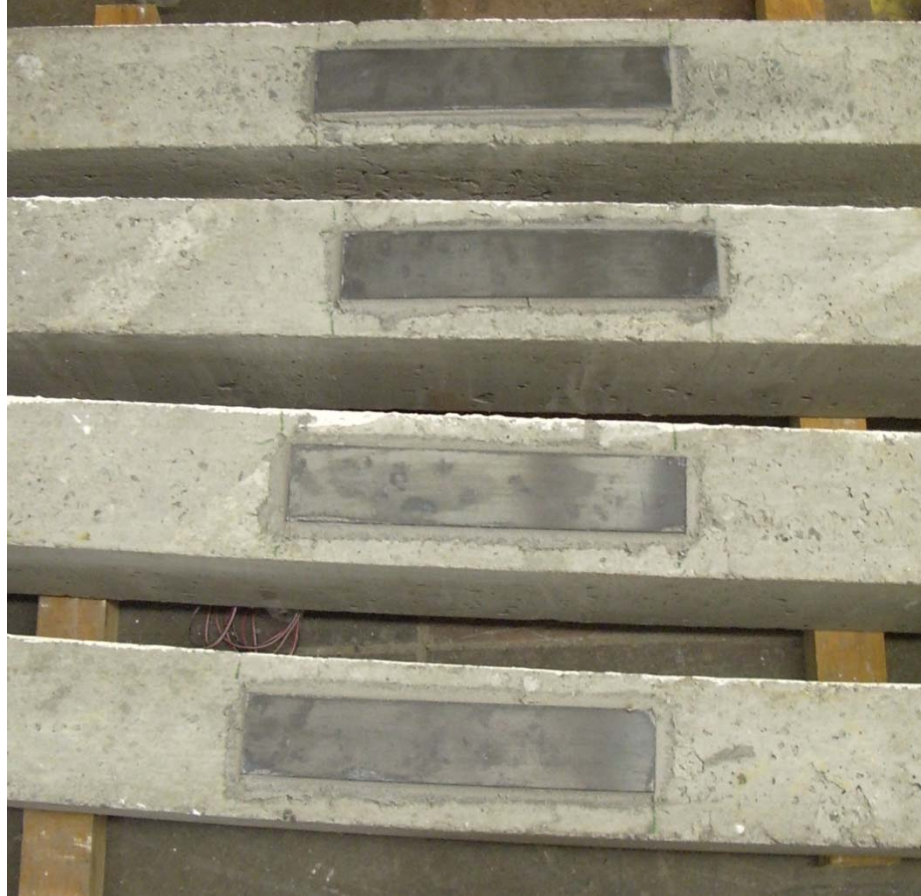
Figure G.3. Flexural reinforced beam repaired with CarboDur patches.
