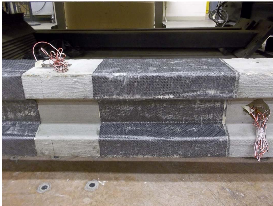
Figure G.5. View of bonded composite U-jacket repair of PSCB3 beam.
