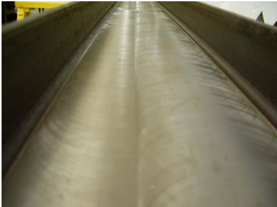
Figure D.4. A view of web of beam SBII after milling [63].
