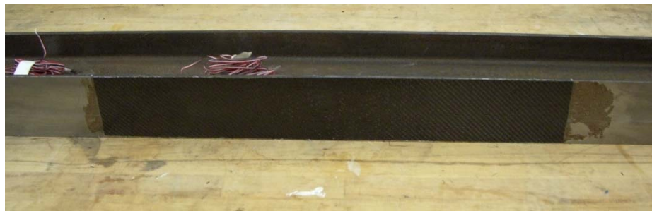
Figure G.1. Steel beam repaired with prepreg FRP composite.
