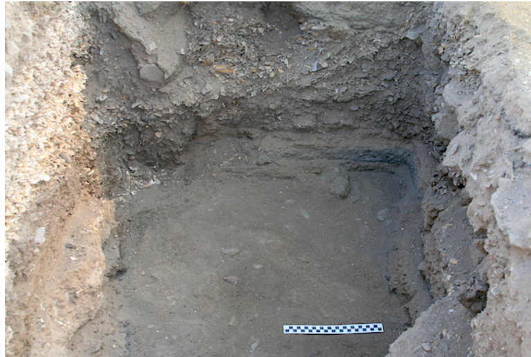
Figure 3.5: Profile of south wall in sector A3. The south and west profiles were unstable, with a risk of collapsing.
