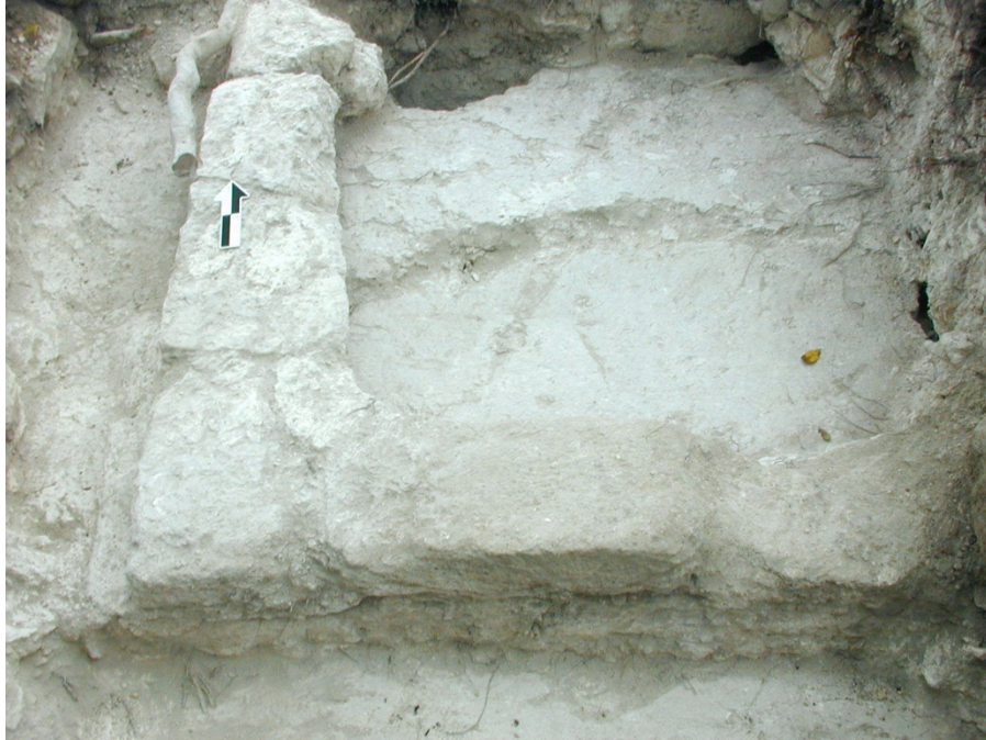
Figure 4.43 Foundation walls of Late Classic residence constructed on top of Structure 1 (photo by the author)
