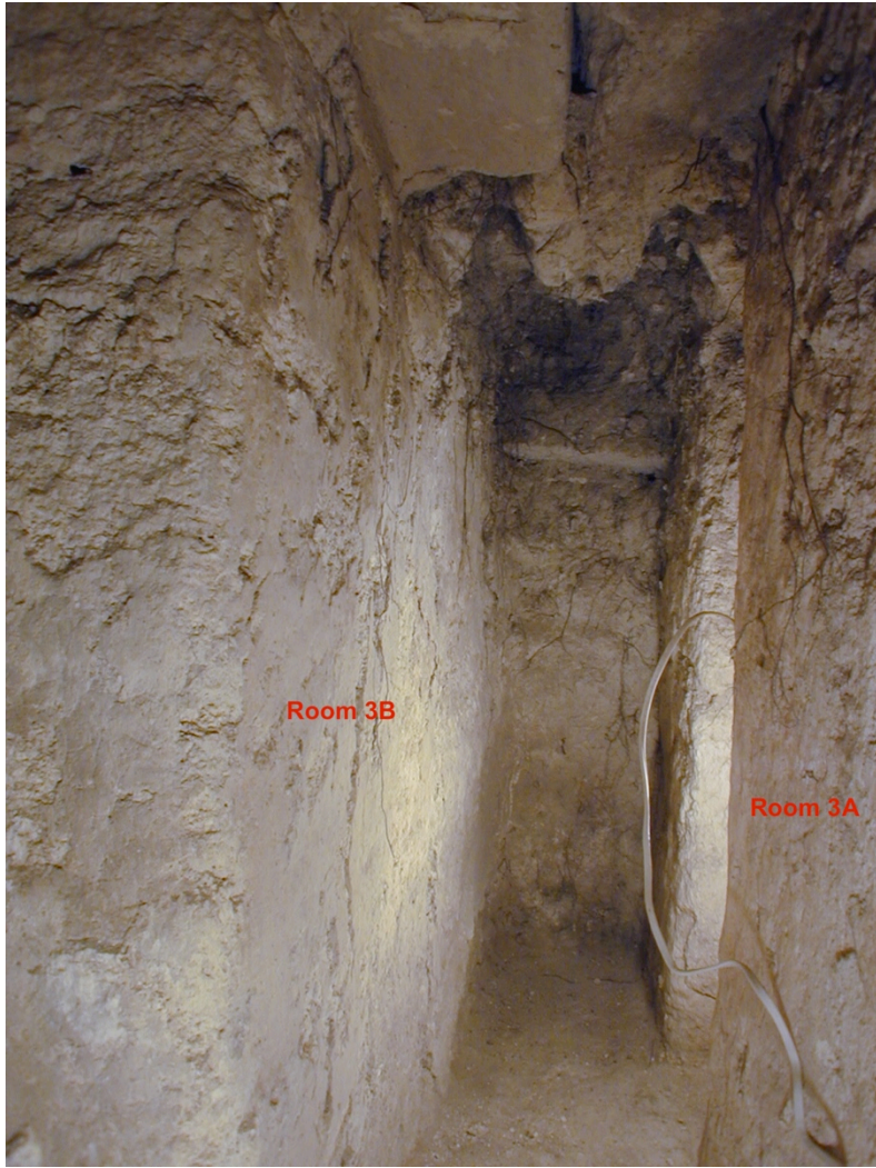
Figure 4.26 Interface of Room 3A, wall ST17.43, and Room 3B. Note the floor of Room 3A continues seamlessly from the interior of the room to the passage between the two rooms (photo by the author)
