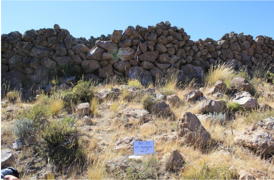
Figure B.13. Exterior of the defensive wall.
