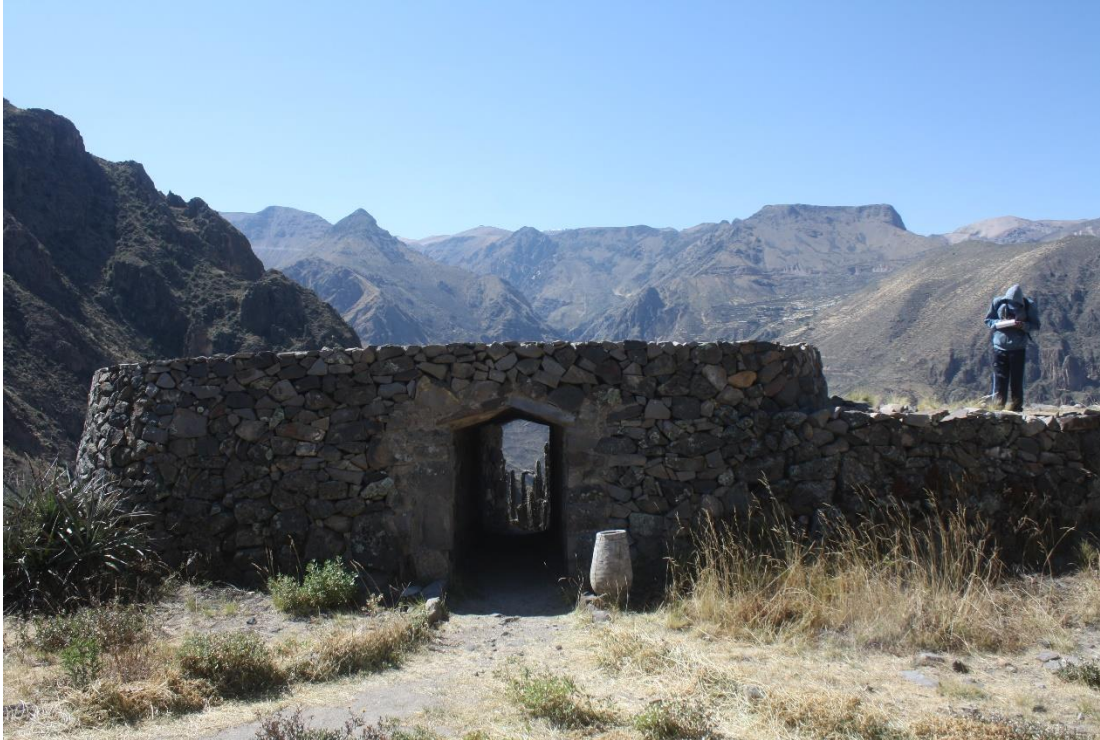
Figure B.120. Reconstructed access to the site.
