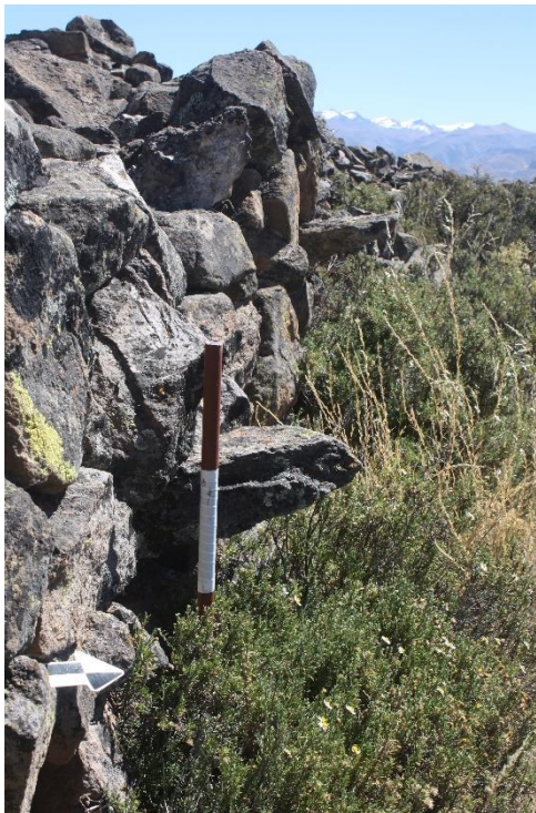
Figure B.14. Talons along the interior of defensive wall.
