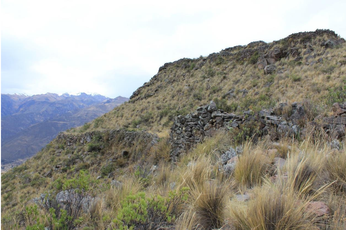
Figure B.111. View of the defensive walls on the western side of the hilltop.
