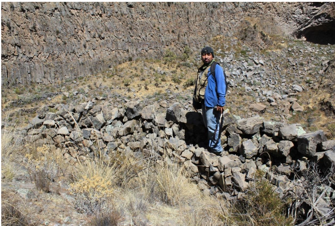
Figure B.95. Wall parapet.
