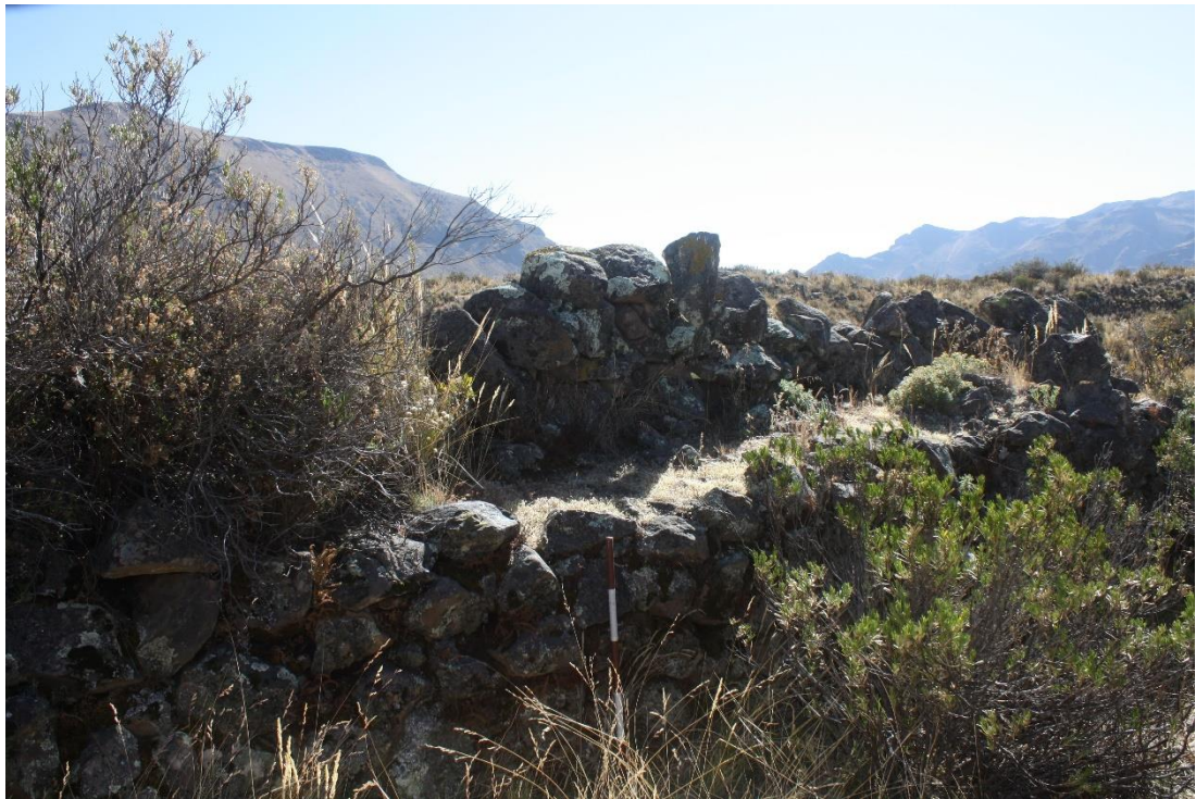
Figure B.159. Parapet on the interior of the wall.
