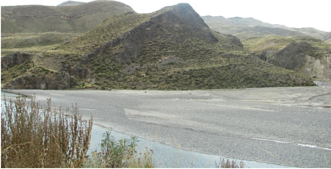
Figure B.47. View of CA-203 from the north.
