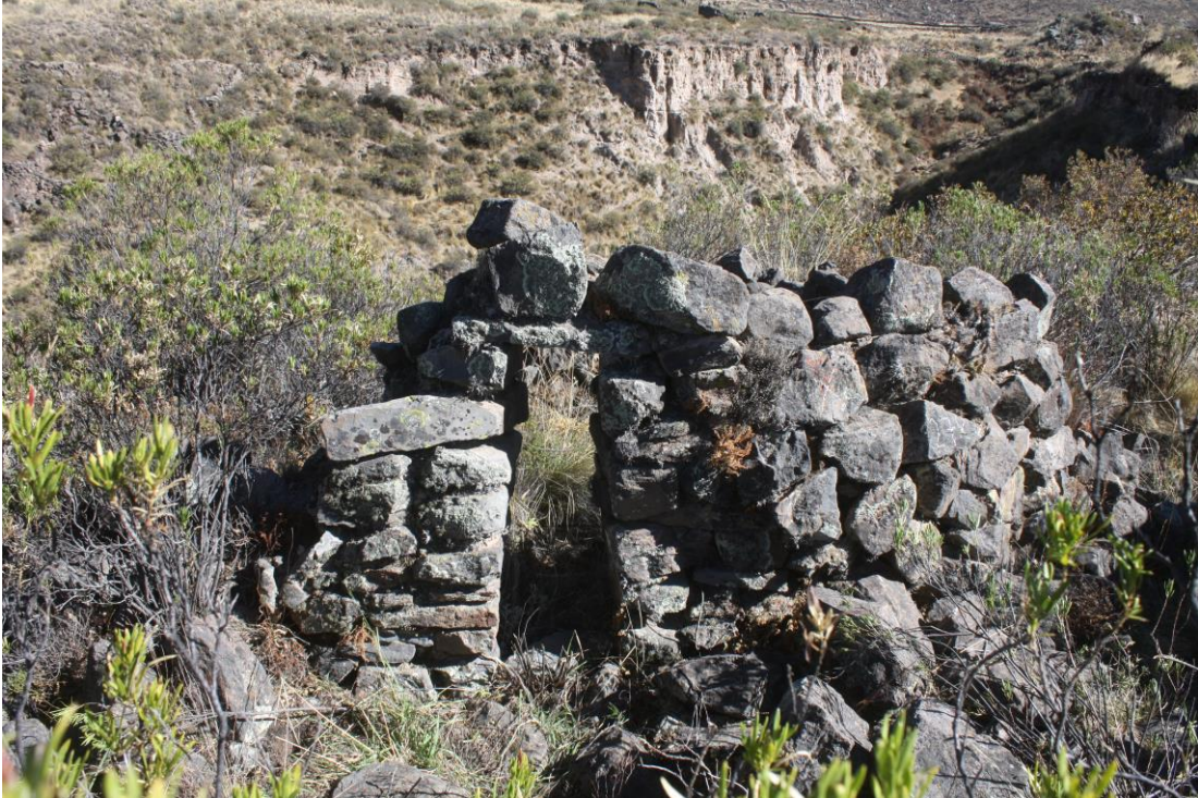
Figure 6.1. Example of a circular structure with well-preserved doorway.
