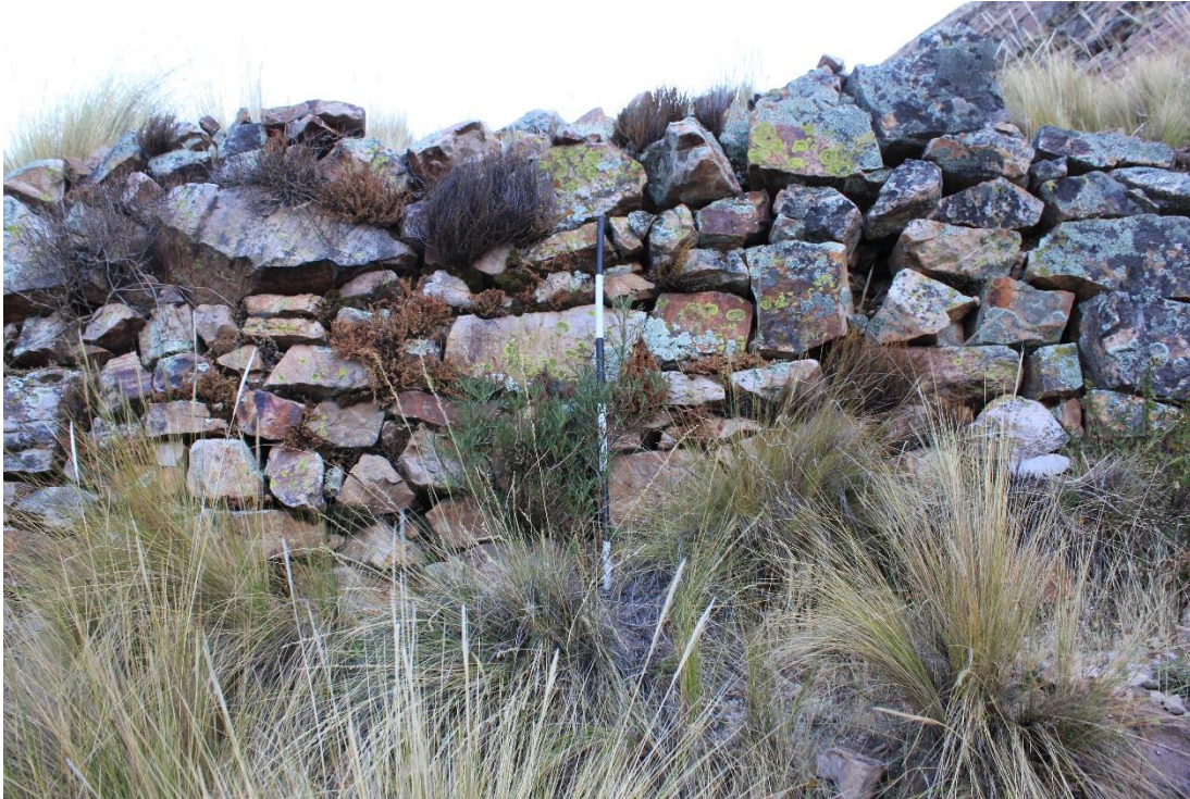
Figure B.131. Exterior of defensive wall.
