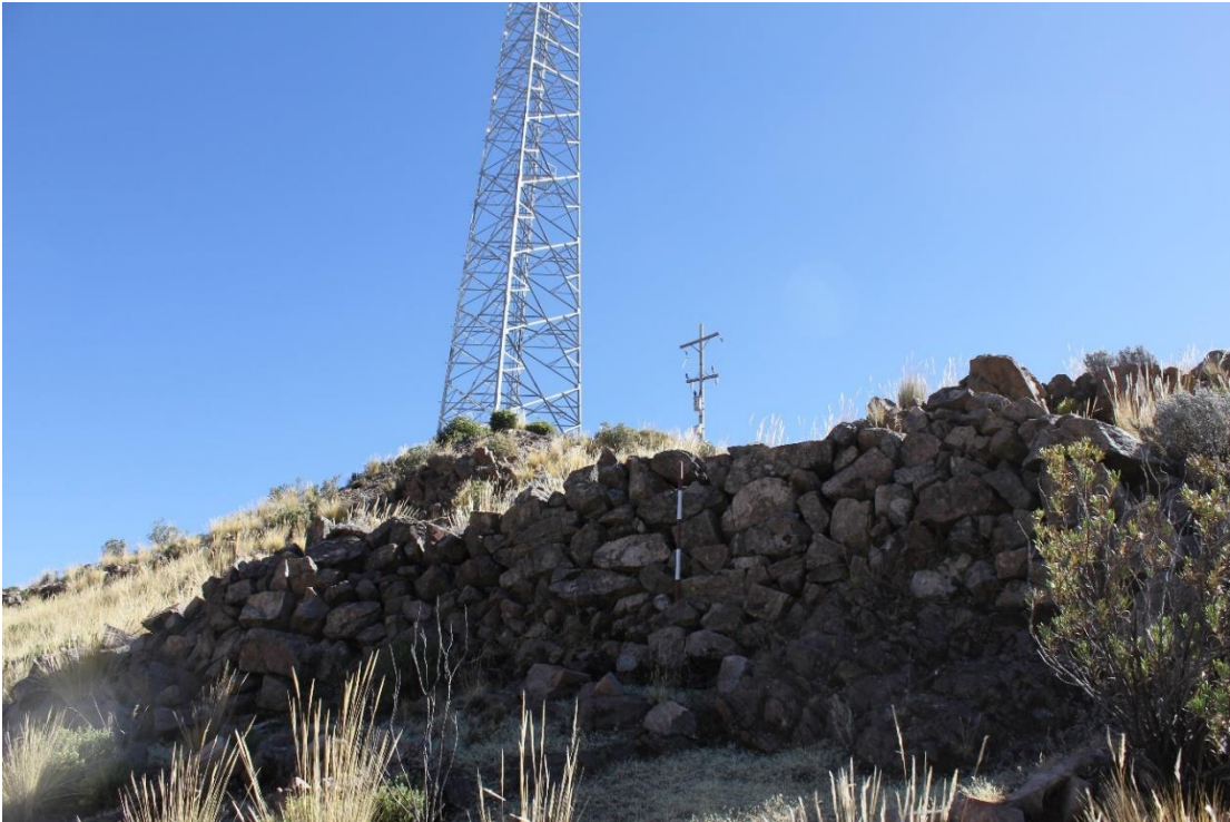
Figure B.61. Exterior of defensive wall.
