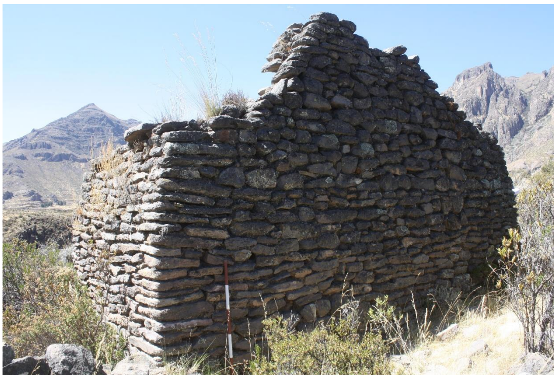
Figure B.161. High status domestic structure in Sector I.
