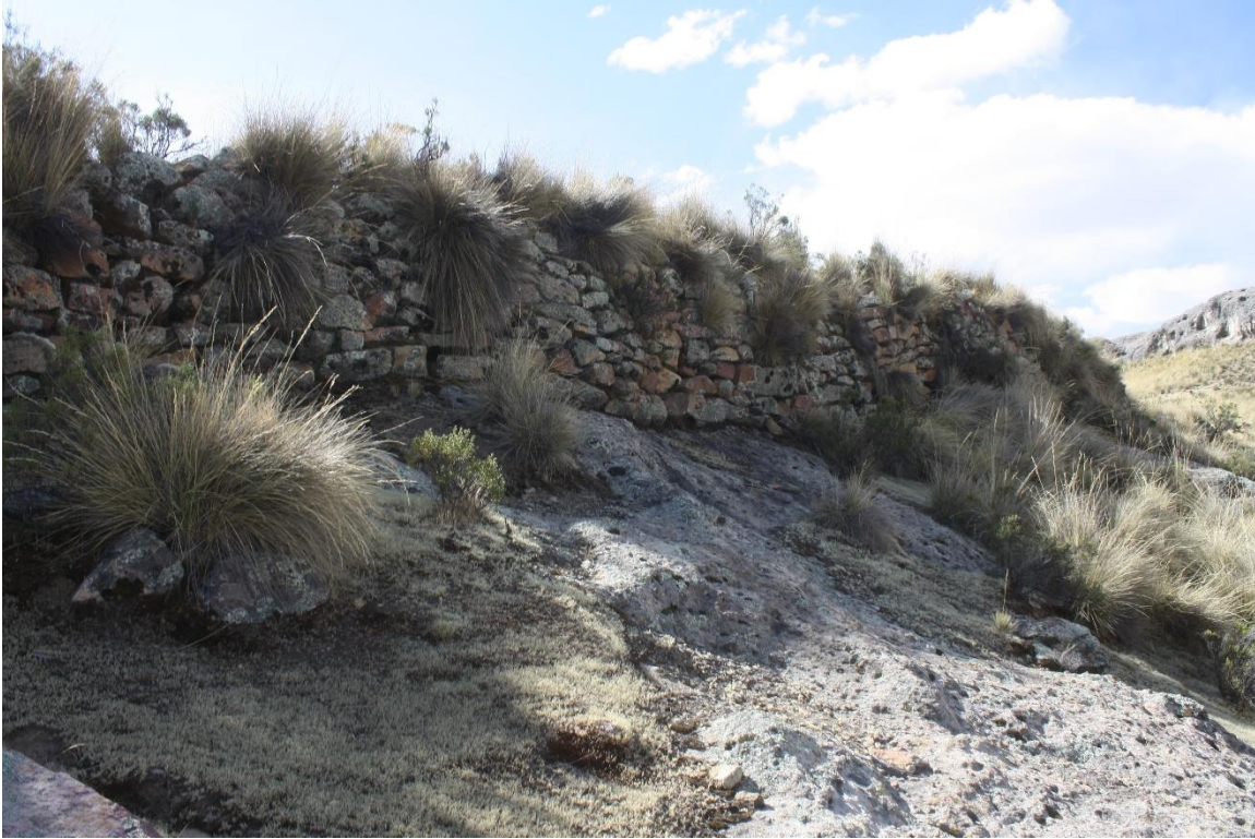
Figure B.28. Exterior side of one of the defensive walls.
