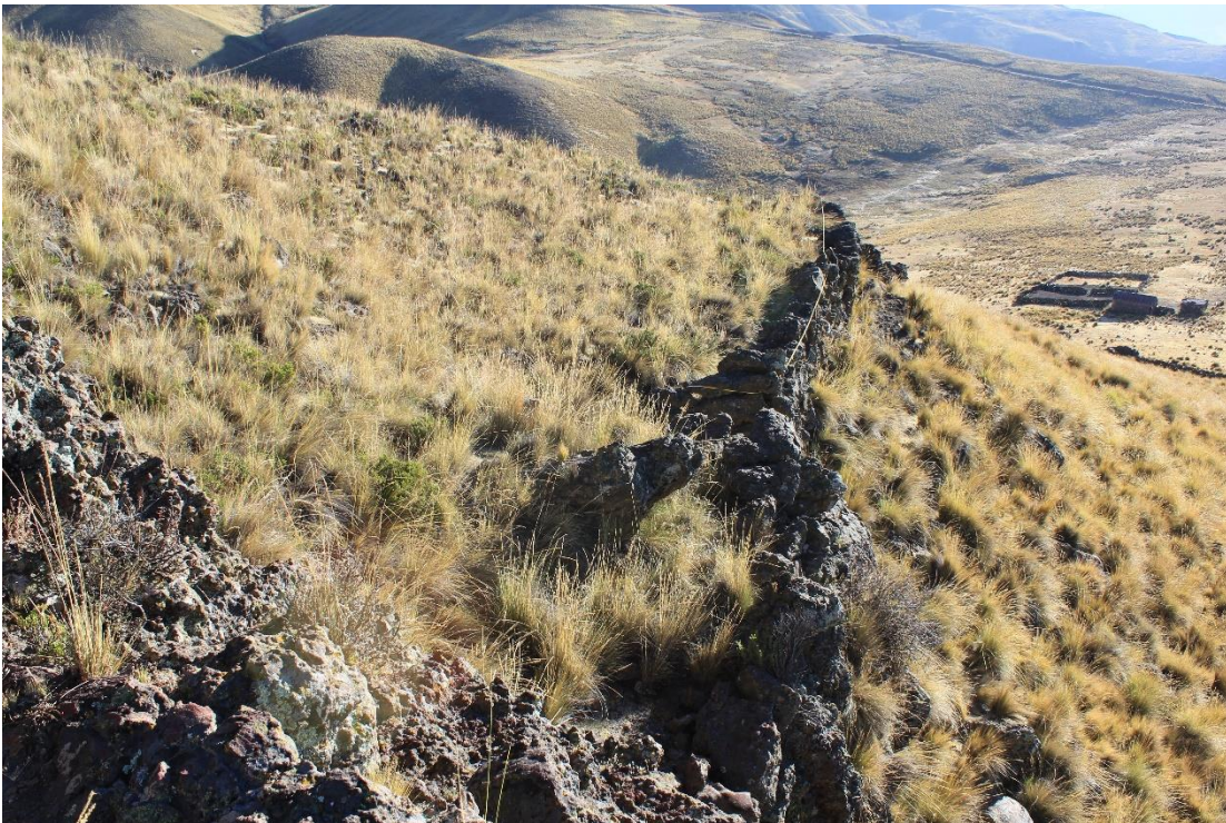
Figure B.134. Outer defensive wall.
