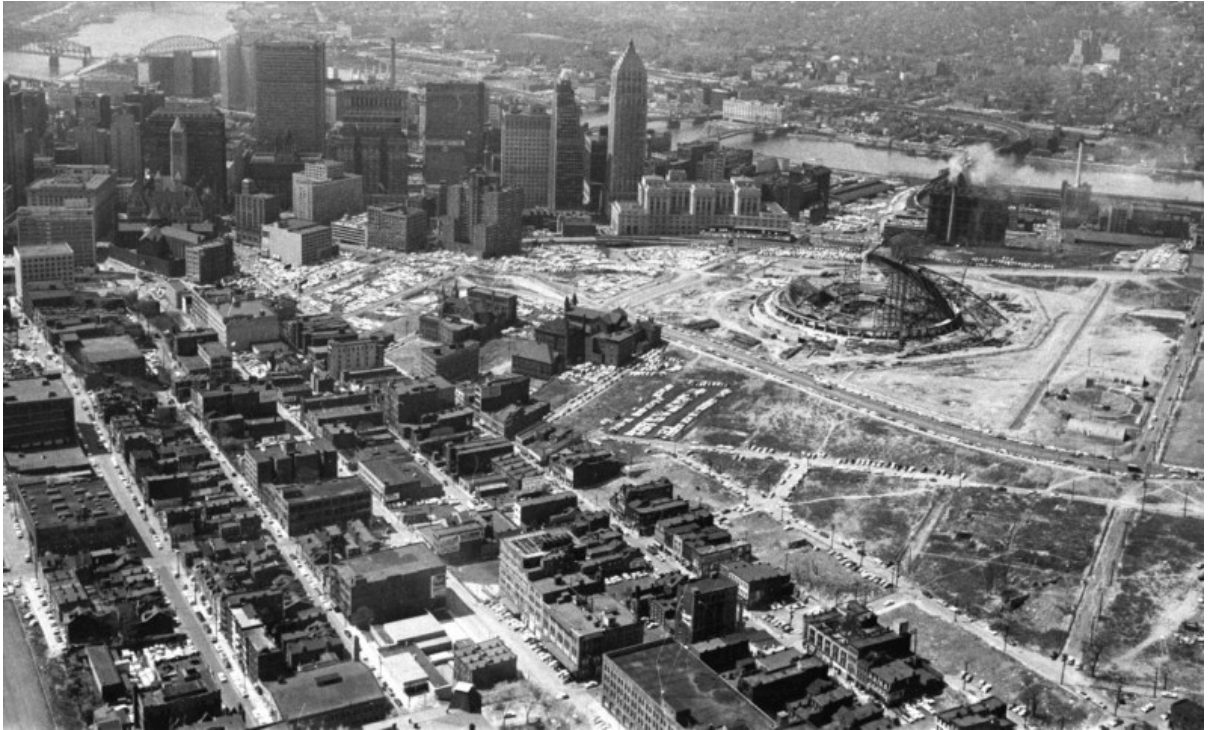
Figure 26 Construction of Civic Arena, ca. 1960s
