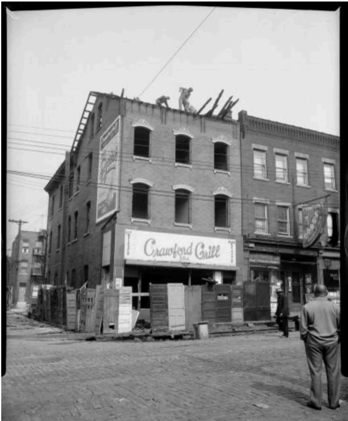
Figure 31 Charles “Teenie” Harris, Workers Demolishing Roof of Crawford Grill No. 1 , 1956, photograph
