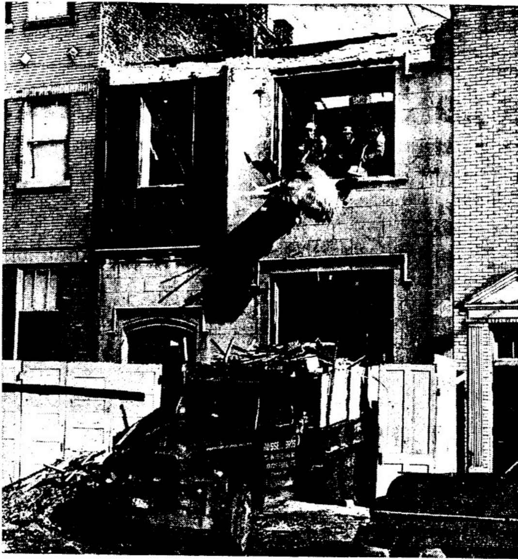
Wreckers demolish three story building at 1251 N. La Salle st. as first stage in slum clearance project on near north side by Chicago Land Clearance commission. Entire project will cost estimated 30 million dollars. (TRIBUNE Photo)
