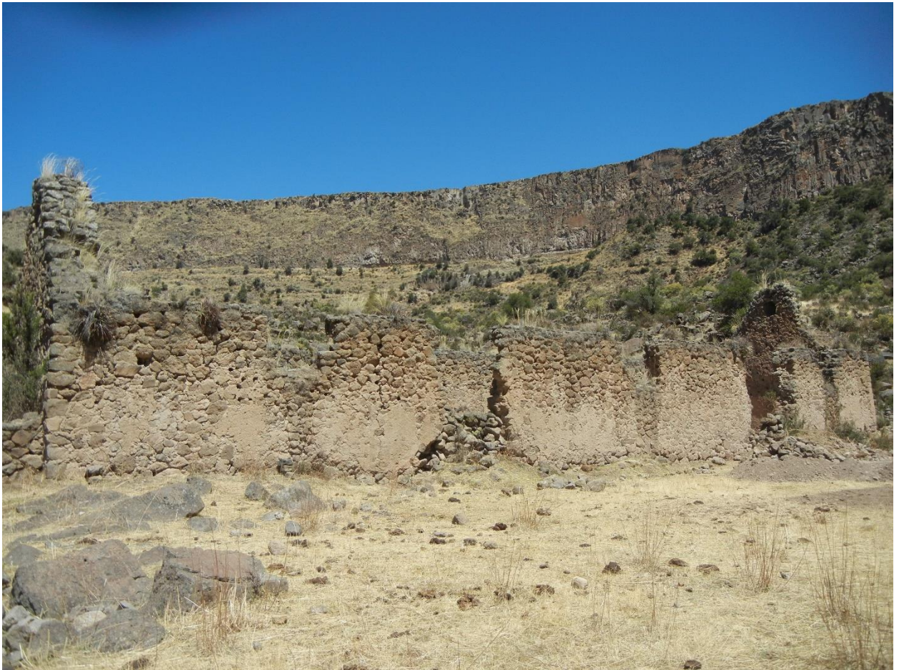
Figure 6.5. Exterior of the northern wall of the church, photo looking south.
