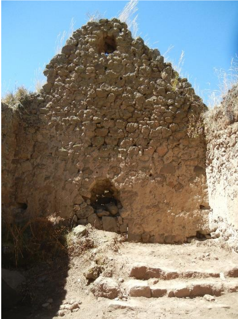
Figure 4.19. Church altar facing east.
