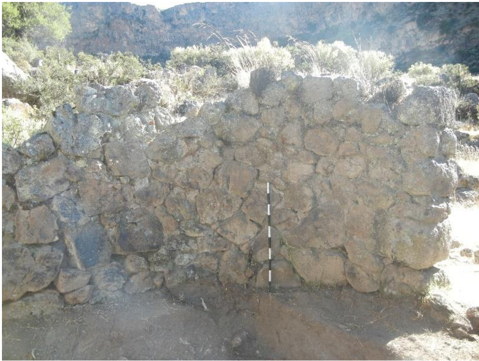
Figure 6.13. Typical uncoursed masonry style with faced stones lining the entrance, photo facing north.
