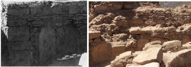
**Figure 7.2** Images of wall masonry at La Galgada (left; Grieder et al 1988, Figure 52) and Perolcoto (right; structure PC-A) show how, at both sites, the wall foundations were constructed with large upright stones that were surrounded by small chinking stones.
