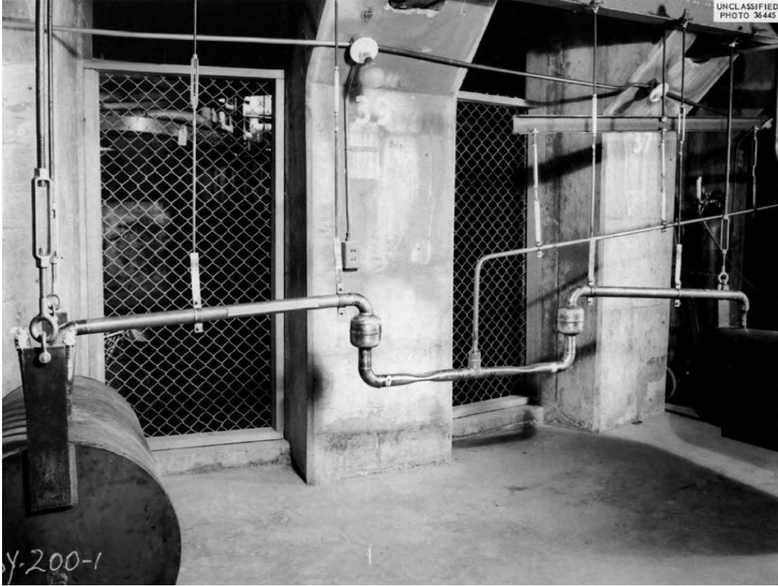
Figure 18: Example of freeze valve piping [Briggs, 1961]
