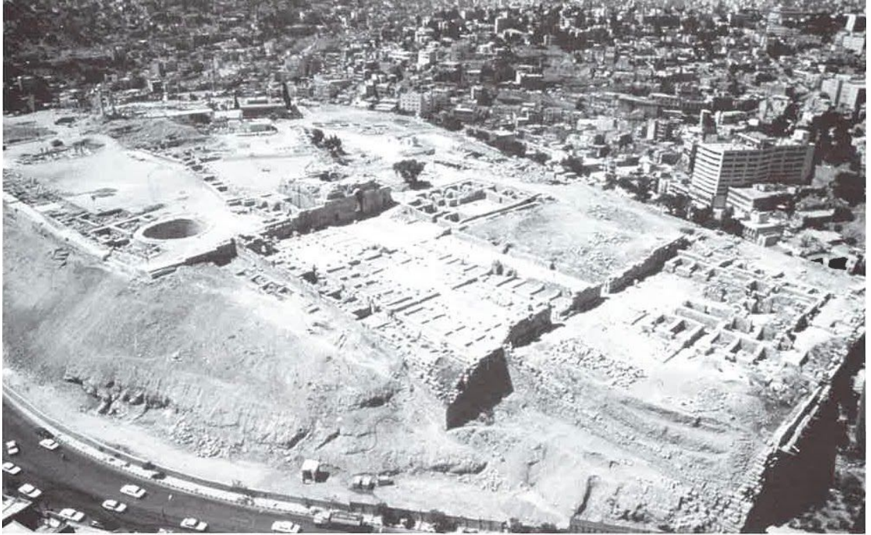
Figure 74: General view of the Umayyad citadel at Amman. Almagro, El palacio omeya de Amman , 301.
