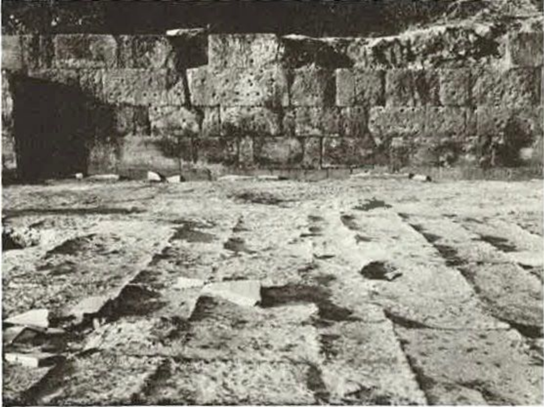
Figure 76: Palace wall from al-Walid's Minya palace near Tiberias, with visible pitting in the stone wall for the purpose of installing marble panelling. Creswell, EMA , plate 67f.
