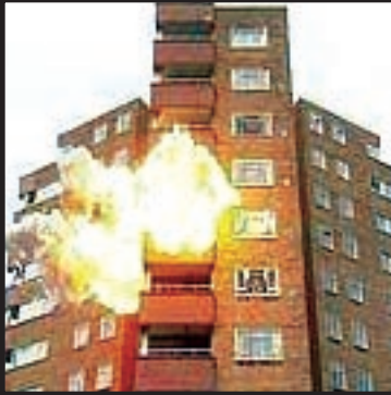
Result of Module Failures
